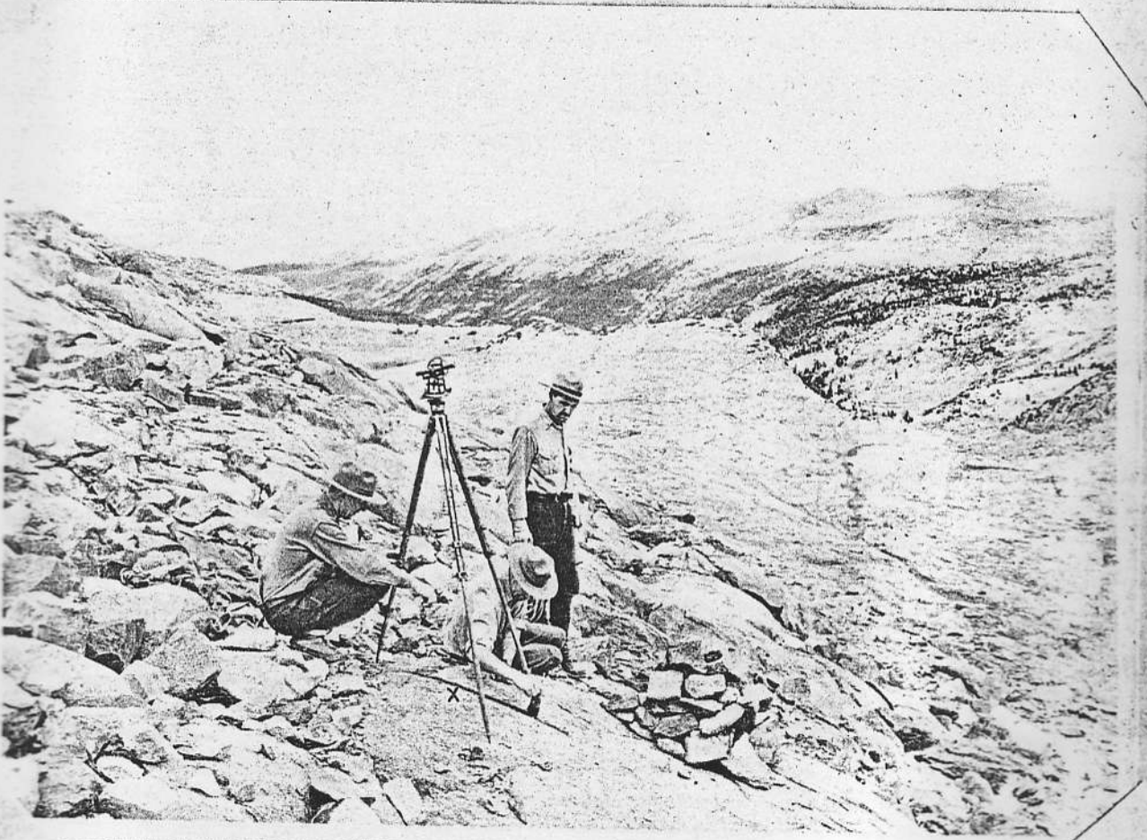
The end points X and Y of the base line just described we marked with green paint on the native granite. We also built monuments to make these reference points more easily found for future measurements. This photo, looking north, shows the glaciated canyon of the Lyell Fork of the Tuolumne River.
